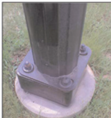
Duratel light pole installed on legacy base
