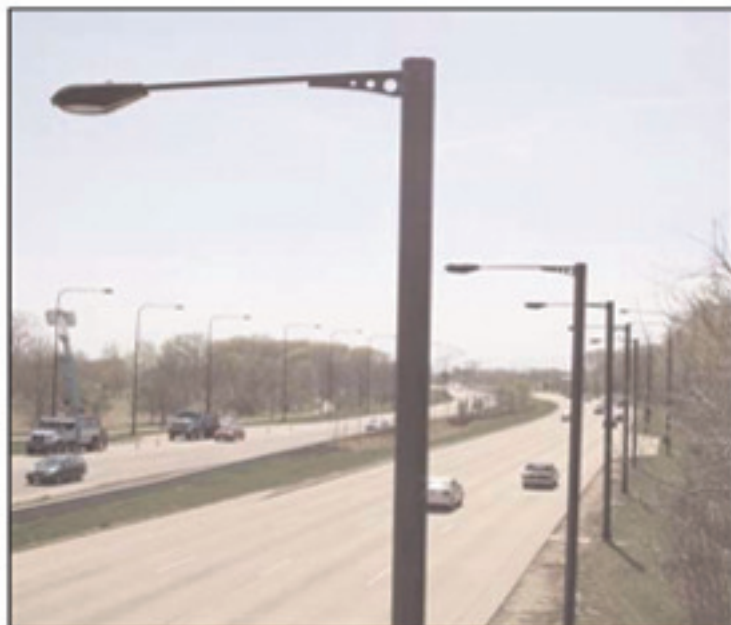
Lake Shore Drive installation looking south
